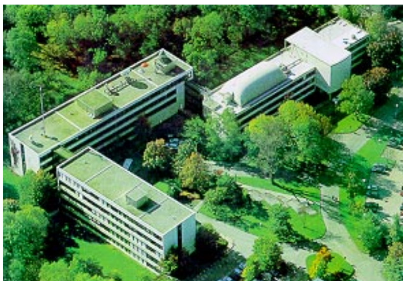
Figure 1 Aerial view of the IRT, Munich.
