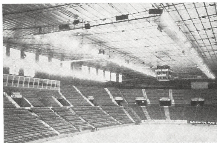
Overall view of the stadium showing the three lighting gantries. (Sveriges Radio photo)
