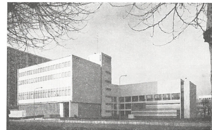
Fig. 2. — The east front of the new Lyons Broadcasting House. Left: Television Block. Right: Sound Block. (Yves Godard, Lyons, photo)
