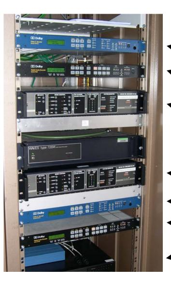
Example of an 5.1 audio installation in a TV broadcast environment.
