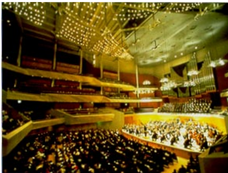
Figure 8 Bridgewater Hall, Manchester (opened 1996, 2400 seats). A hybrid design with sparsely-populated side tiers whose soffits work with the side walls to serve as “2 nd -order” lateral reflectors.
