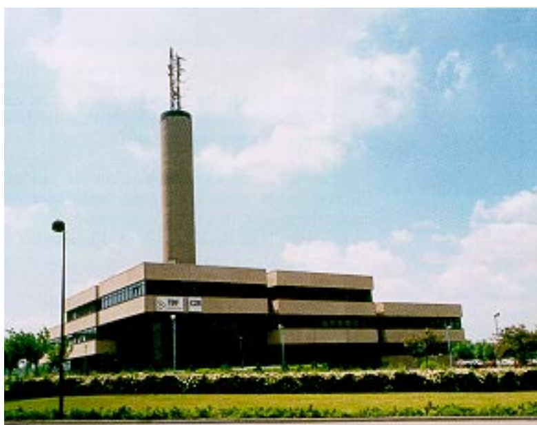
Figure 4 General view of TDF-C2R, Metz.
