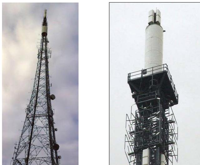
Figure G3: Craikelly tower (left) and top section showing FM arrays (right)
