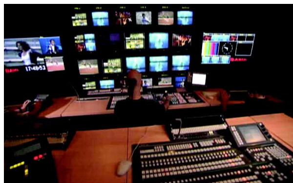
Figure 3 The spacious production area with the monitor wall.
