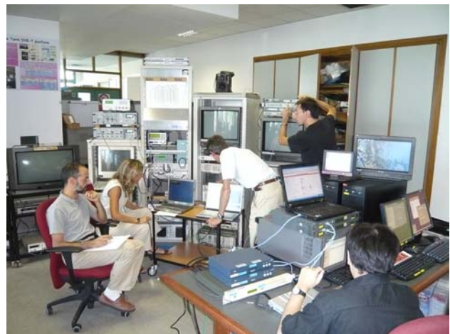
Figure 9 Transmission site in Turin
