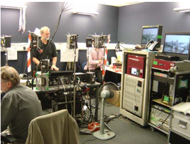
Figure 8 Transmission site in London
