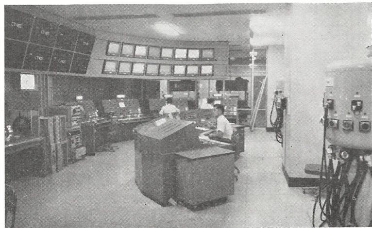
Fig. 4. — The Technical Operation Centre in the new N.H.K. Broadcasting Centre in Tokyo.
