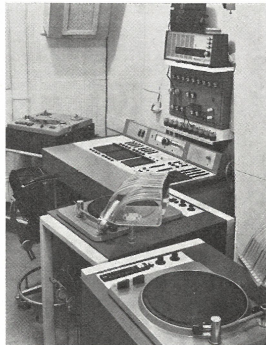
Fig. 3. — The equipment installed in the control room.
