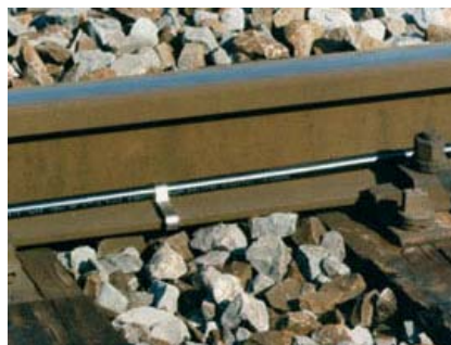
Figure 2 Principle of the Euroloop application (Source: Siemens)
