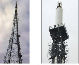
Figure G3: Craigkelly tower (left) and top section showing FM arrays (right)
